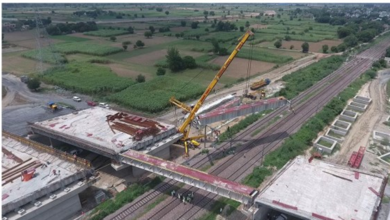
Exhibit 32- Railways Over Bridge
